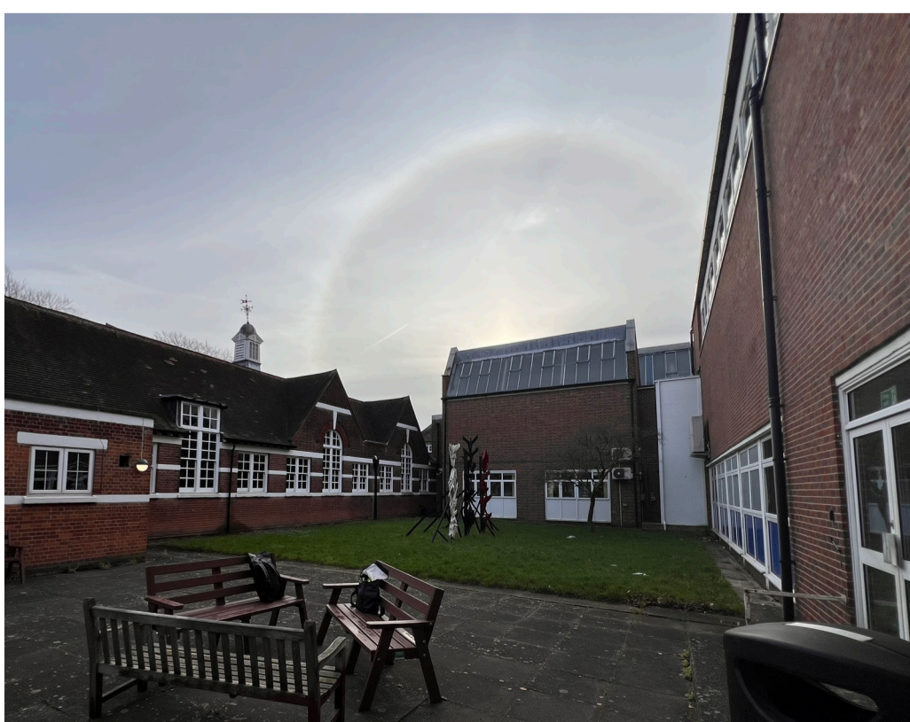
EXISTING COURTYARD AND SITE OF PROPOSED EXTENSION
